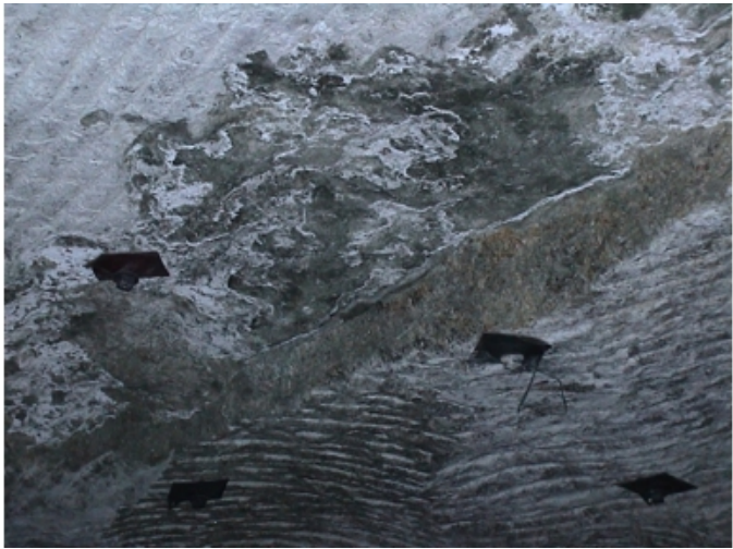
Figure 6.10 Post Depositional Dissolution within the Trona Bed
