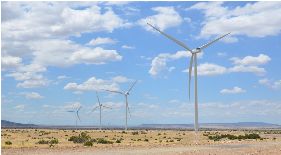
238 MW Chevelon Butte Phase 1 in Arizona, Completed in June 2023
