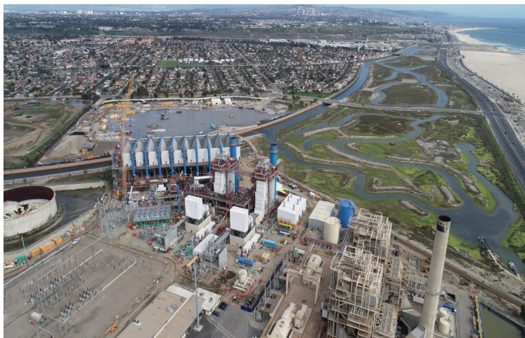
Southland Repowering in California
