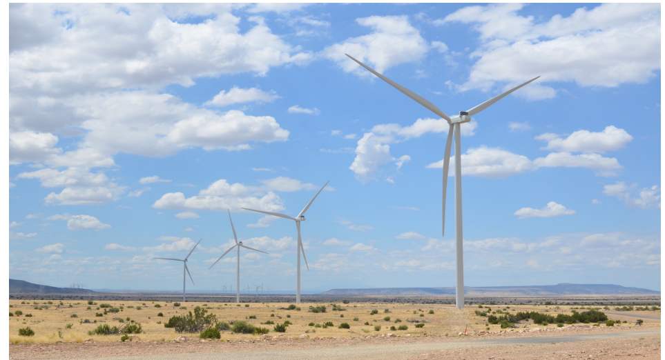
238 MW Chevelon Butte Phase 1 in Arizona
