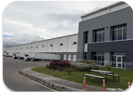
March 2026 Colombia In-country Distribution Center
