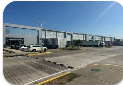
October 2023 Panama Domestic Distribution Center
