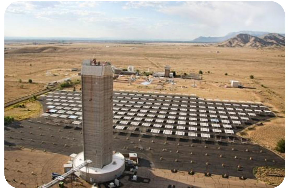
National Solar Thermal Test Facility
