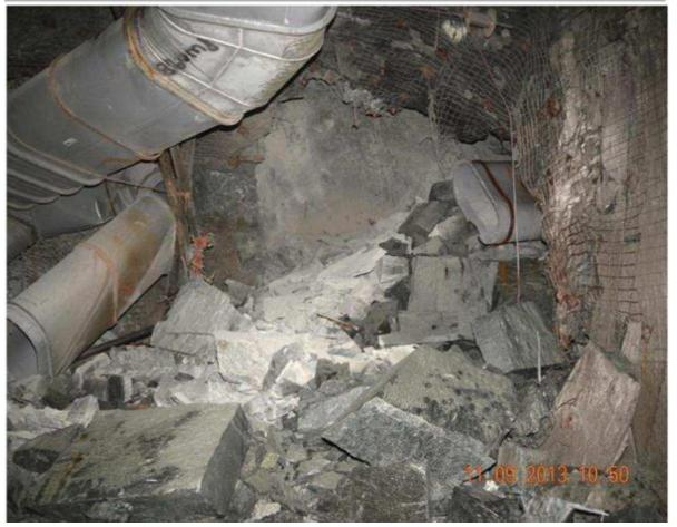
104-07 Level. View looking South from the crosscut access into the 104-07 Level intersection. Appearance is of a Gravity-Induced Fall of Ground, because of the large angular blocks and wedges. Only a few broken support elements can be seen – e.g. remains of a Splitset in the far wall, and 2 broken rebars that can be seen in the centre of the photo.
