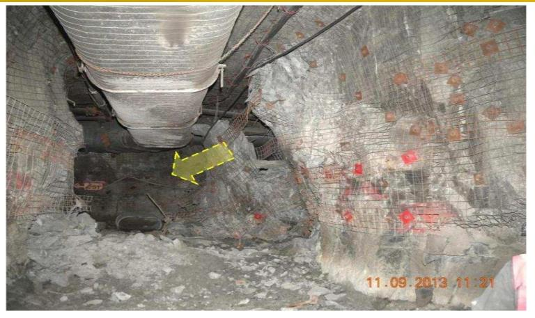
View looking South from the crosscut access into the Level intersection. The Pillar on the right of the photo gives the appearance of having failed suddenly, ejecting the rock laterally into the drift as shown. The back condition is relatively good – damage is to the West wall only. This pillar failure is the likely cause of the gravity induced FOGs on Level 104-08, Level 104-07 and 104-06 below. These intersections are stacked relatively closely above one another.
