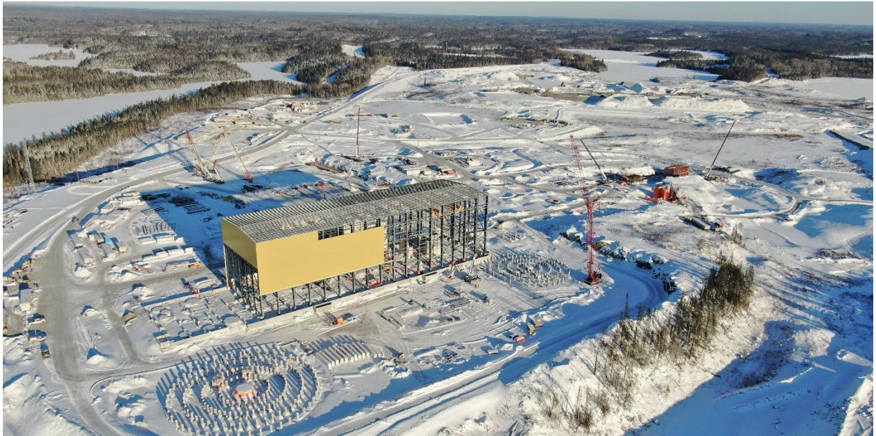
Côte Gold – Processing Plant Wall Panel Cladding (January 2022)
