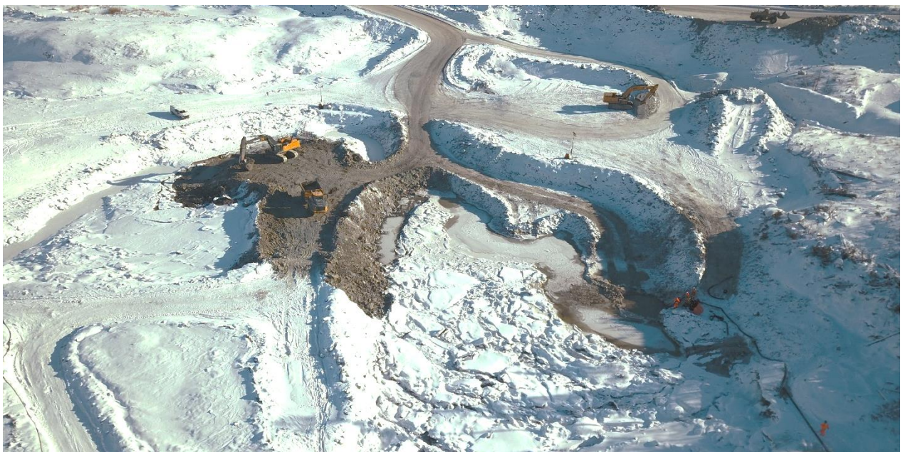
Côte Gold – TMF Starter Dam Foundation Excavation (January 2022)
