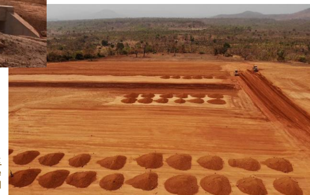
RIGHT: Permanent Camp – Laterite Ready to be Levelled
