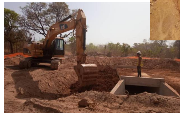
TOP: Box-culvert – Backfill in Progress
