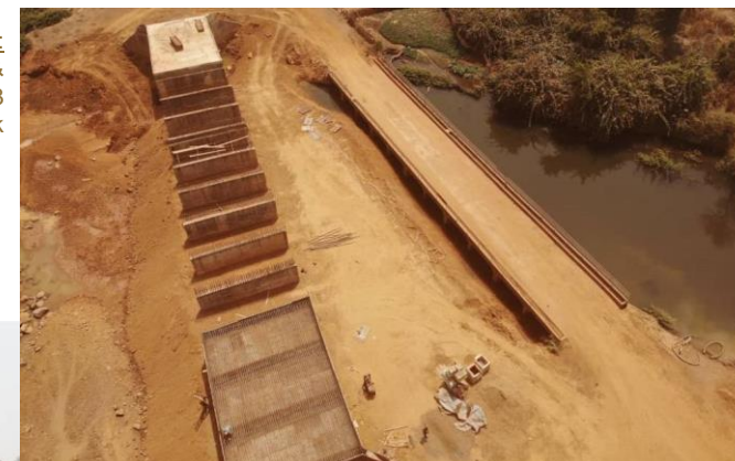
RIGHT: Saroudia Bridge Formwork & Reinforcement in Place on 3 Sections of the Bridge Deck
