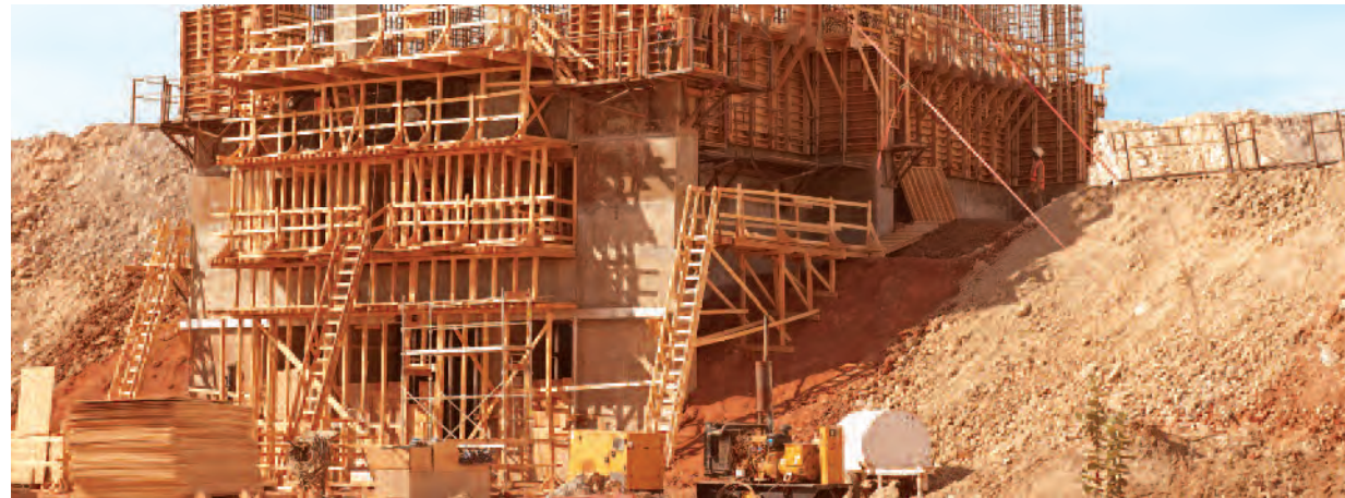
FOUNDATION FOR ESSAKANE CRUSHER
