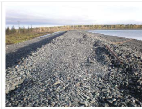
Example of water management structure
