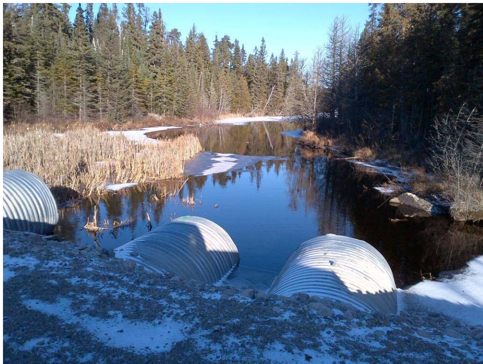
Photograph 25: Côté Outlet Looking Downstream toward Upper Three Duck Lakes
