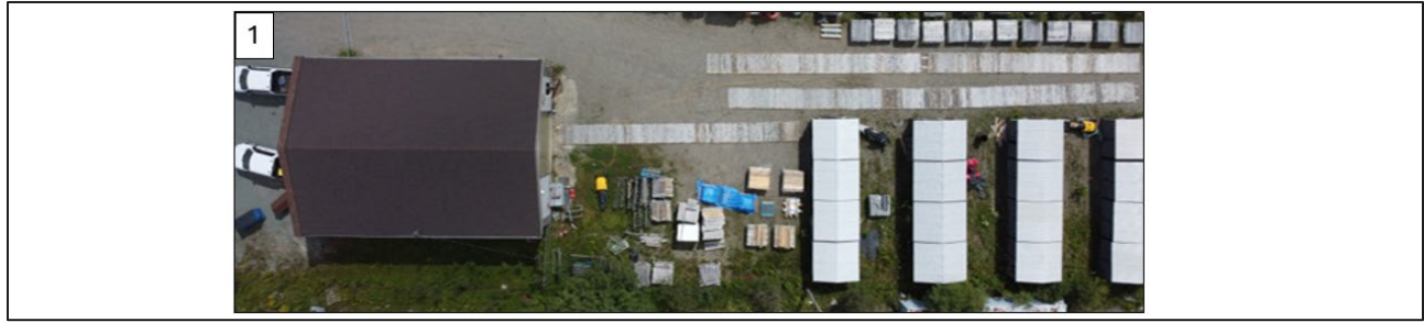
Figure 5-2: Core Shack Facility in Chibougamau
