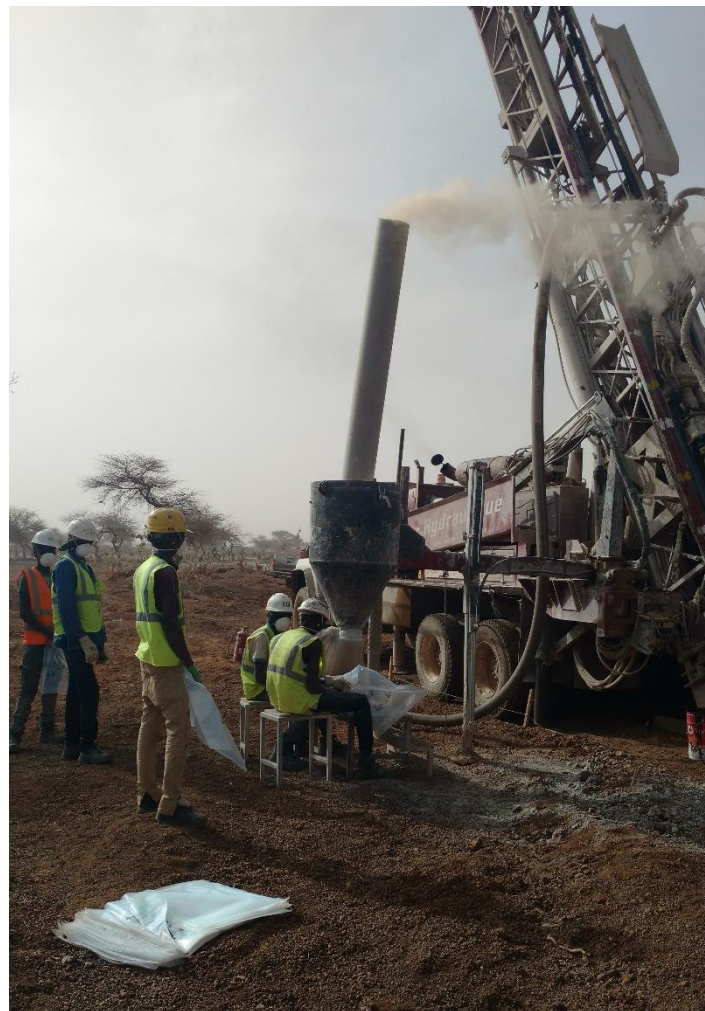
Figure 10.4: Reverse Circulation Drilling at Gossey – March 2018
