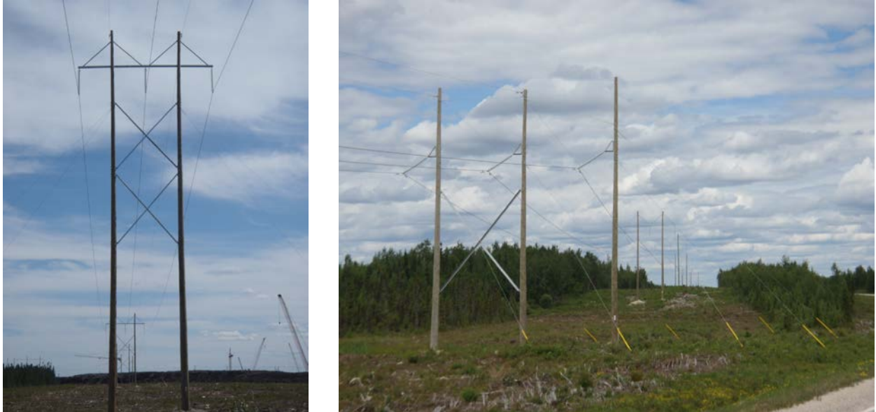
Photograph 1: Typical 230 / 115 kV Transmission Line and Poles
