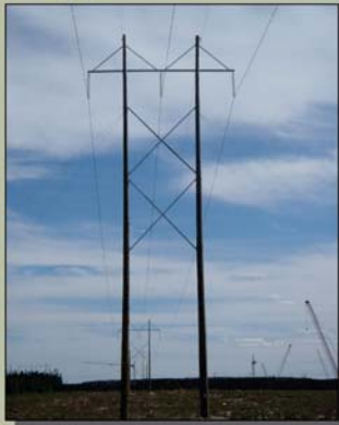
Typical H-Frame Transmission Line and Poles
