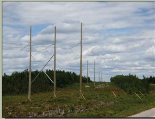
Typical H-Frame Transmission Line and Poles
