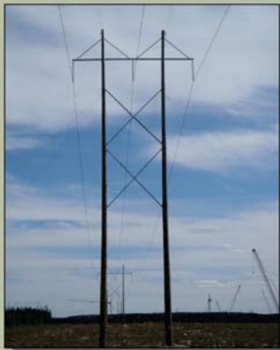
Typical H-Frame Transmission Line and Poles
