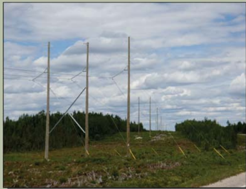
Typical H-Frame Transmission Line and Poles
