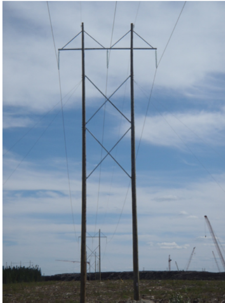
Photograph 4-1: Typical 230 kV Transmission Line and Poles
