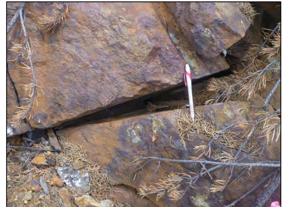
Photo 17: Crevice observed at 100med
