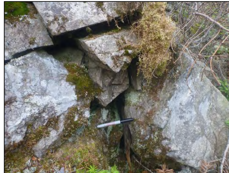
Photo 15: Crevice observed at 117lo
