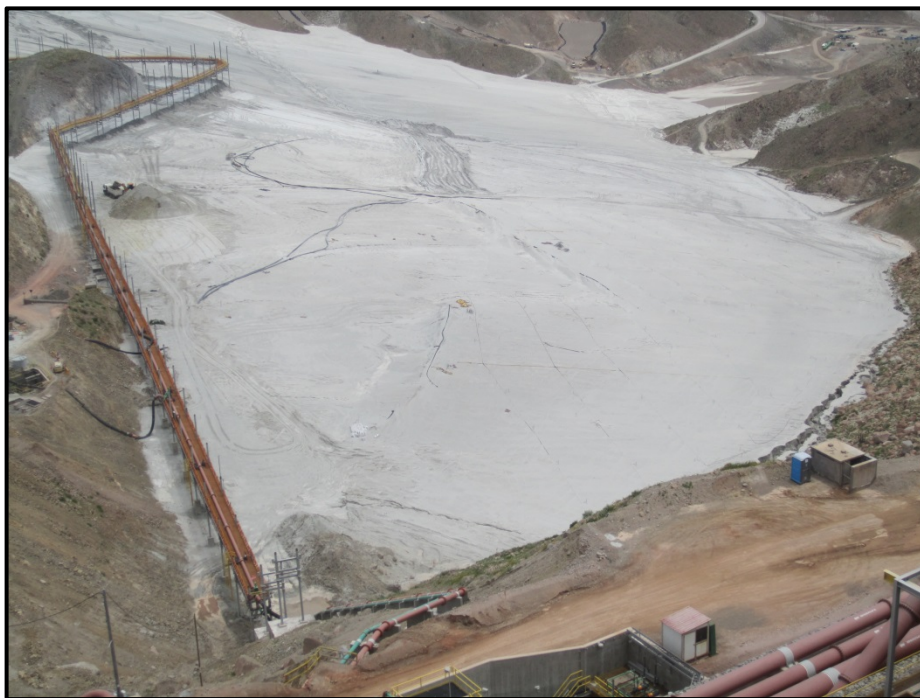
Photograph 1 – Irrigation Dust Control at Cerro Verde Mine
