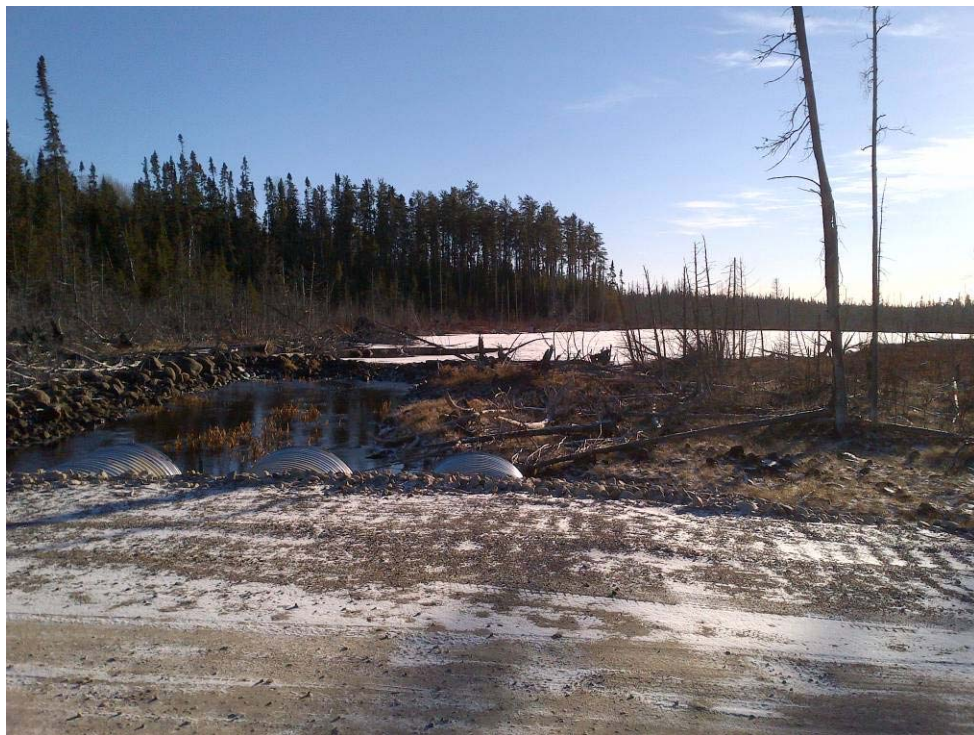
Photograph 16: Chester Lake Outlet Looking Upstream
