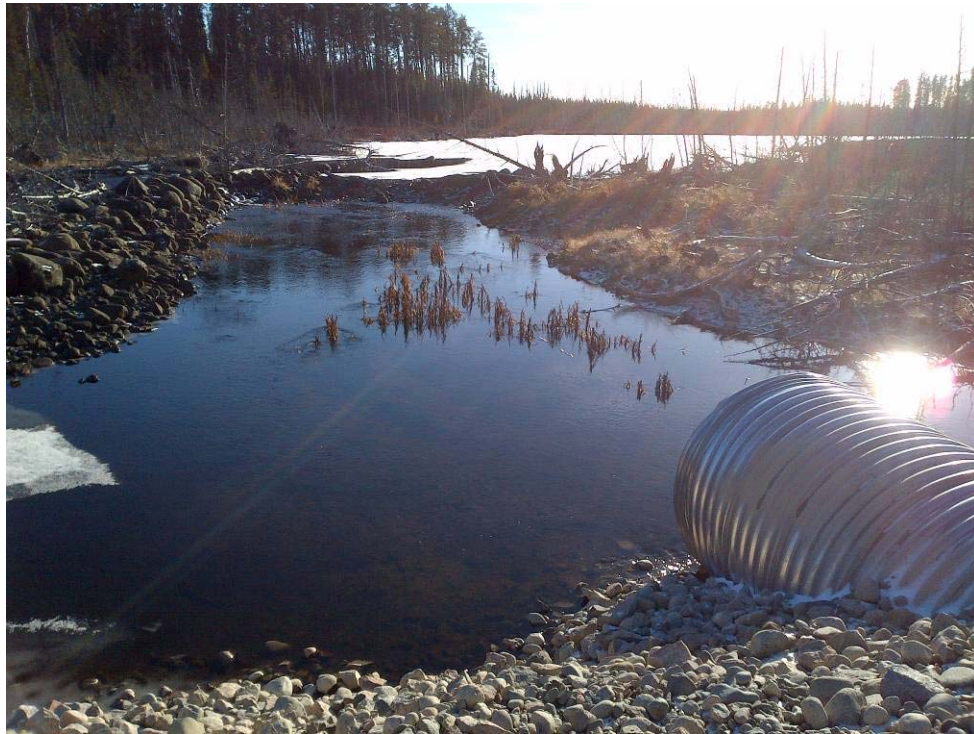
Photograph 15: Chester Lake Outlet Looking Upstream (Looking South)
