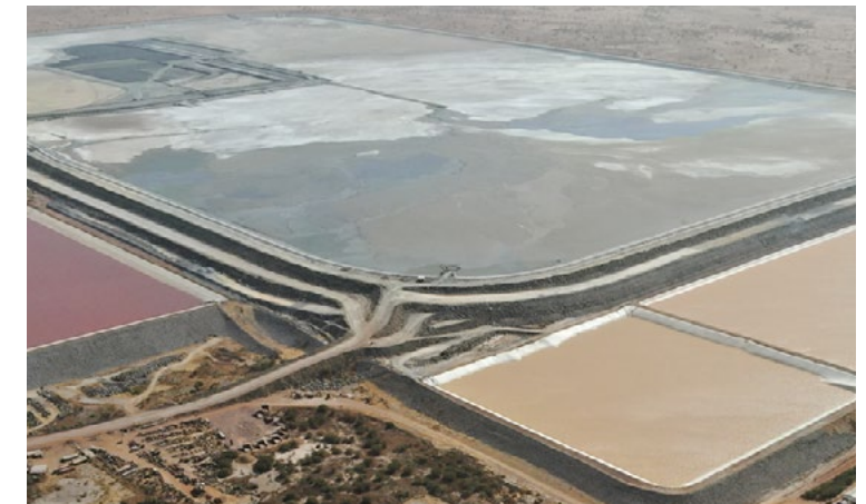
Essakane tailings storage facility
