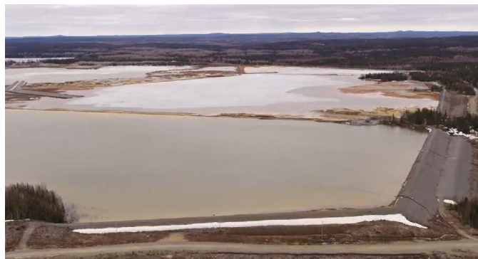
Figure 2: Westwood Tailings Storage Facilities
