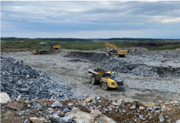
Earthworks – Loading and Hauling
