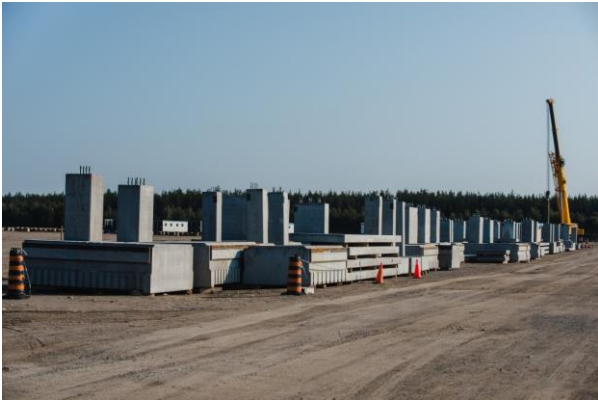
Pre-cast Concrete Foundations
