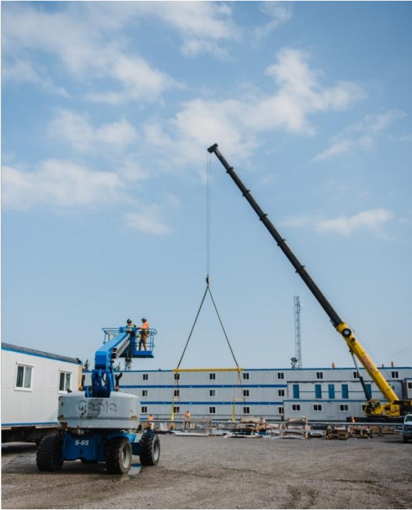
Permanent Camp Construction
