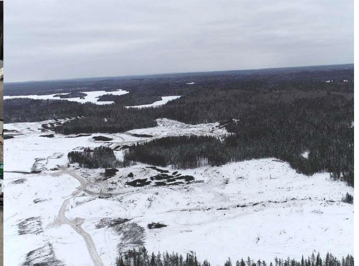
TREE CLEARING – 456 HECTARES COMPLETED
