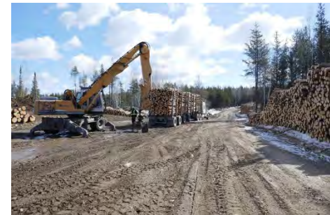
Tree Clearing – Open pit area – first load of timber being loaded and hauled off-site
