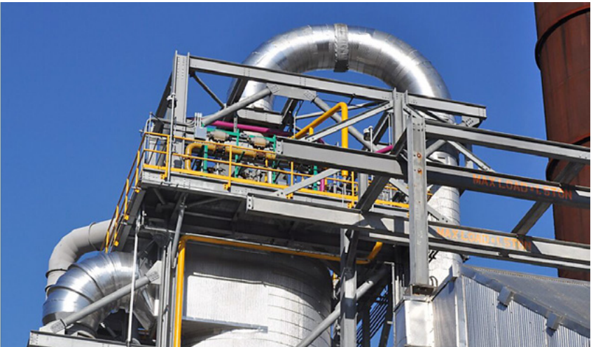
The top of a thermal oxidizer – part of an air emissions control system installed in 2023 at Orion's plant in Belpre, Ohio.
