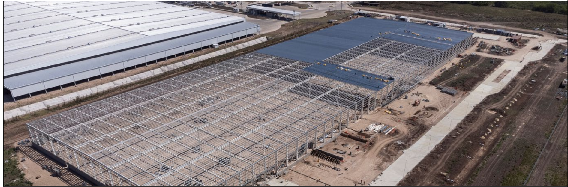
New manufacturing plant under construction in Argentina.
