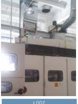
Lodz and Siena implemented a heat recovery system, allowing the re-use of hot air produced by chillers of thermoforming machines and compressors to warm up factory locations and reduce energy use from heating systems.
