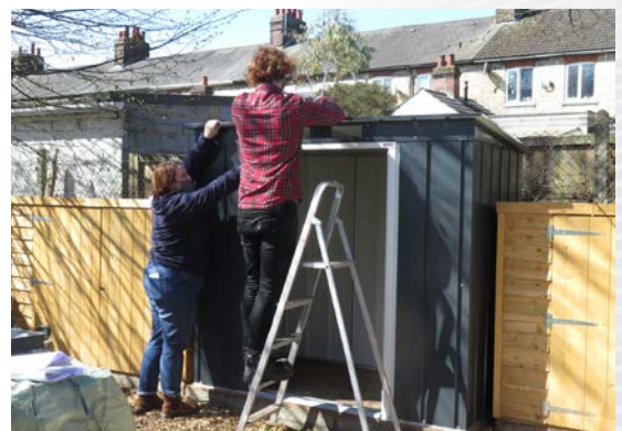
Crane Building Services & Utilities associates in Hitchin, UK, assembling a shed for Triangle Community Garden.
