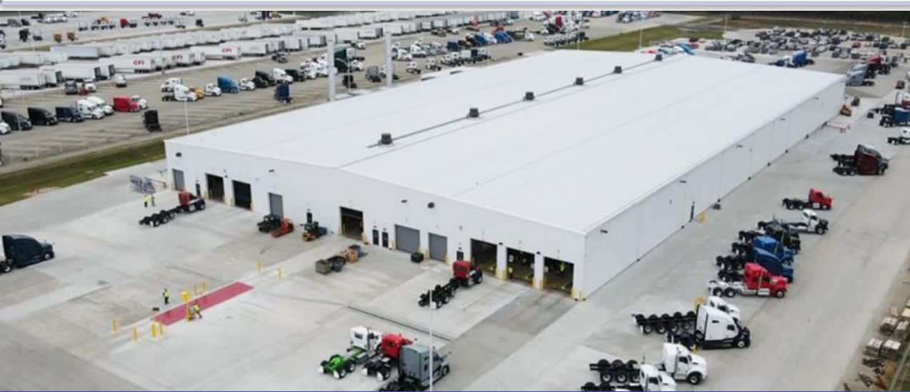
Kenworth New Test Building, Chillicothe, Ohio
