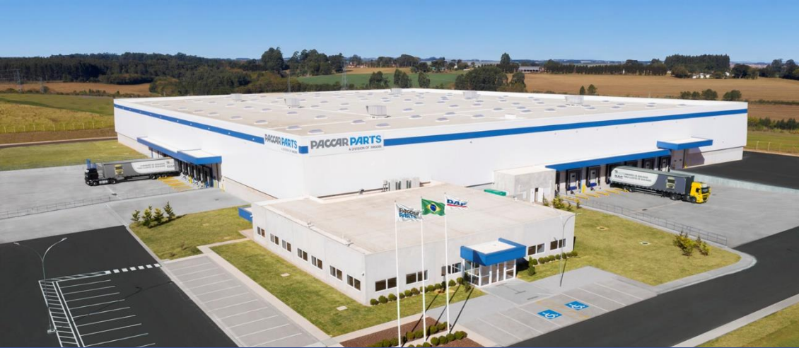
Parts Distribution Center Ponta Grossa, Brasil
