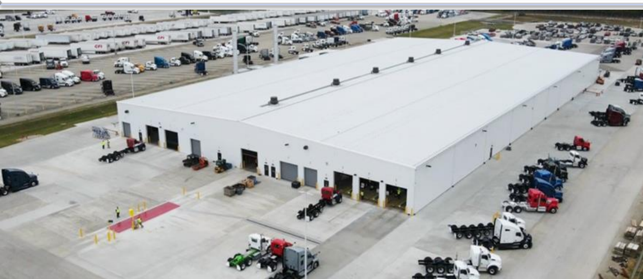
Kenworth New Test Building, Chillicothe, OH
