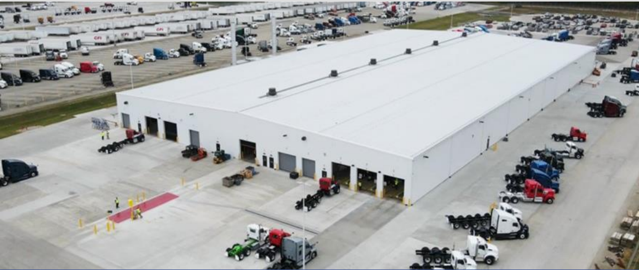
Kenworth New Test Building, Chillicothe, OH
