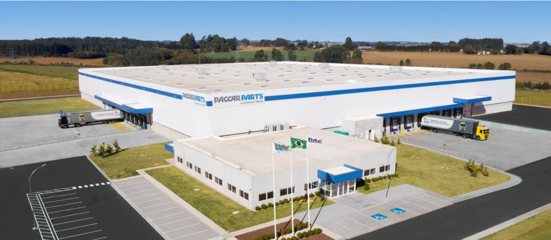
Parts Distribution Center Ponta Grossa, Brasil
