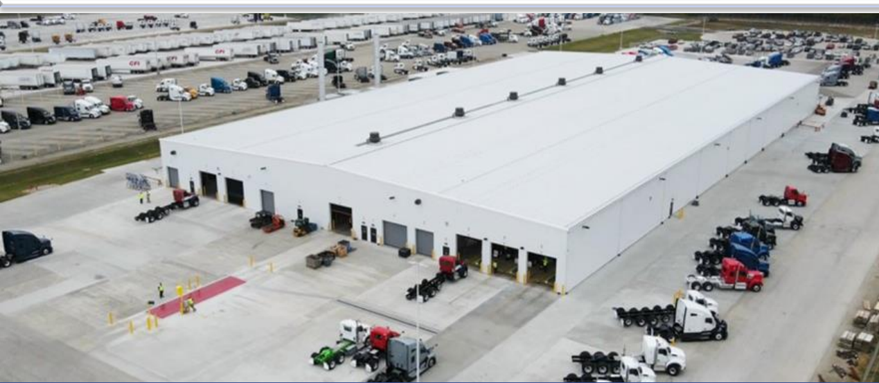
Kenworth New Test Building, Chillicothe, OH
