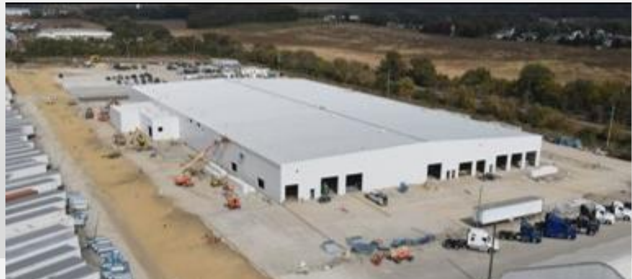
Kenworth New Test Building, Chillicothe, OH
