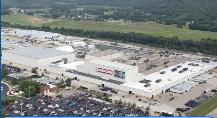
Kenworth Chillicothe Expansion, Ohio
